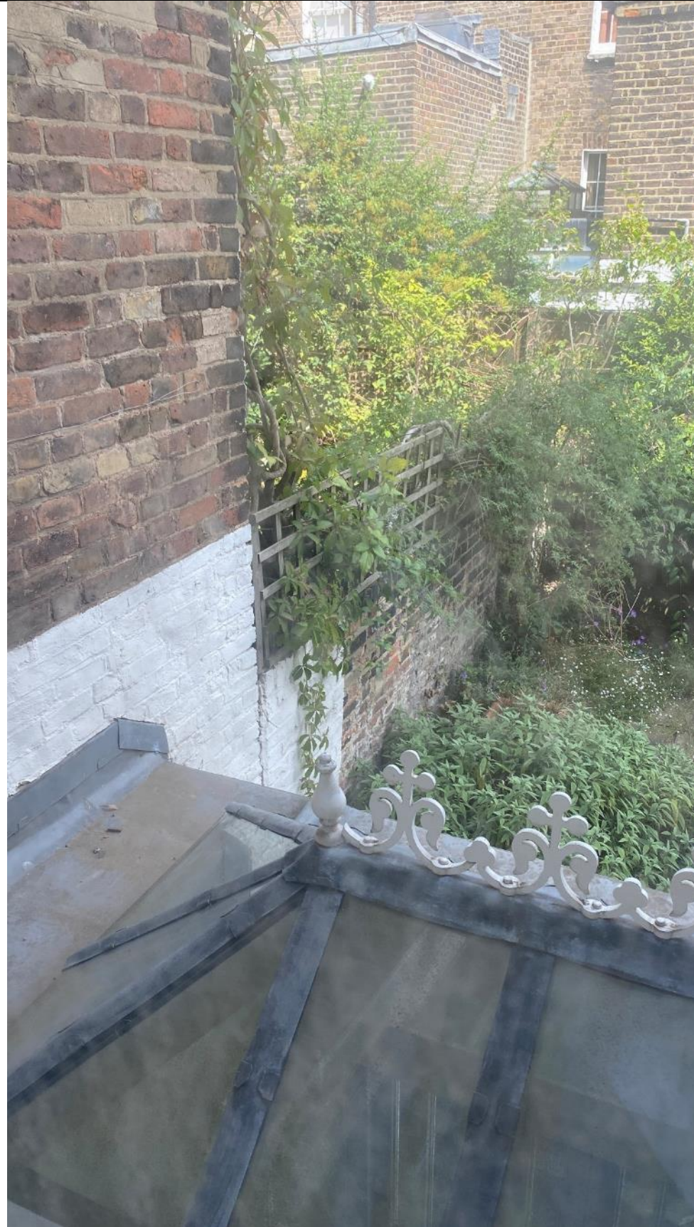
Photo 5: Ground Floor - View outwards of position of new balcony left (north) towards the garden of no.22.
